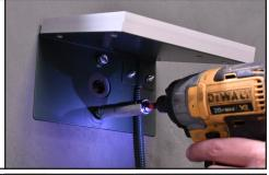
7. Run Solar Charger cable through hole from outside to inside of blind. Sealant is recommended around solar panel cable.
